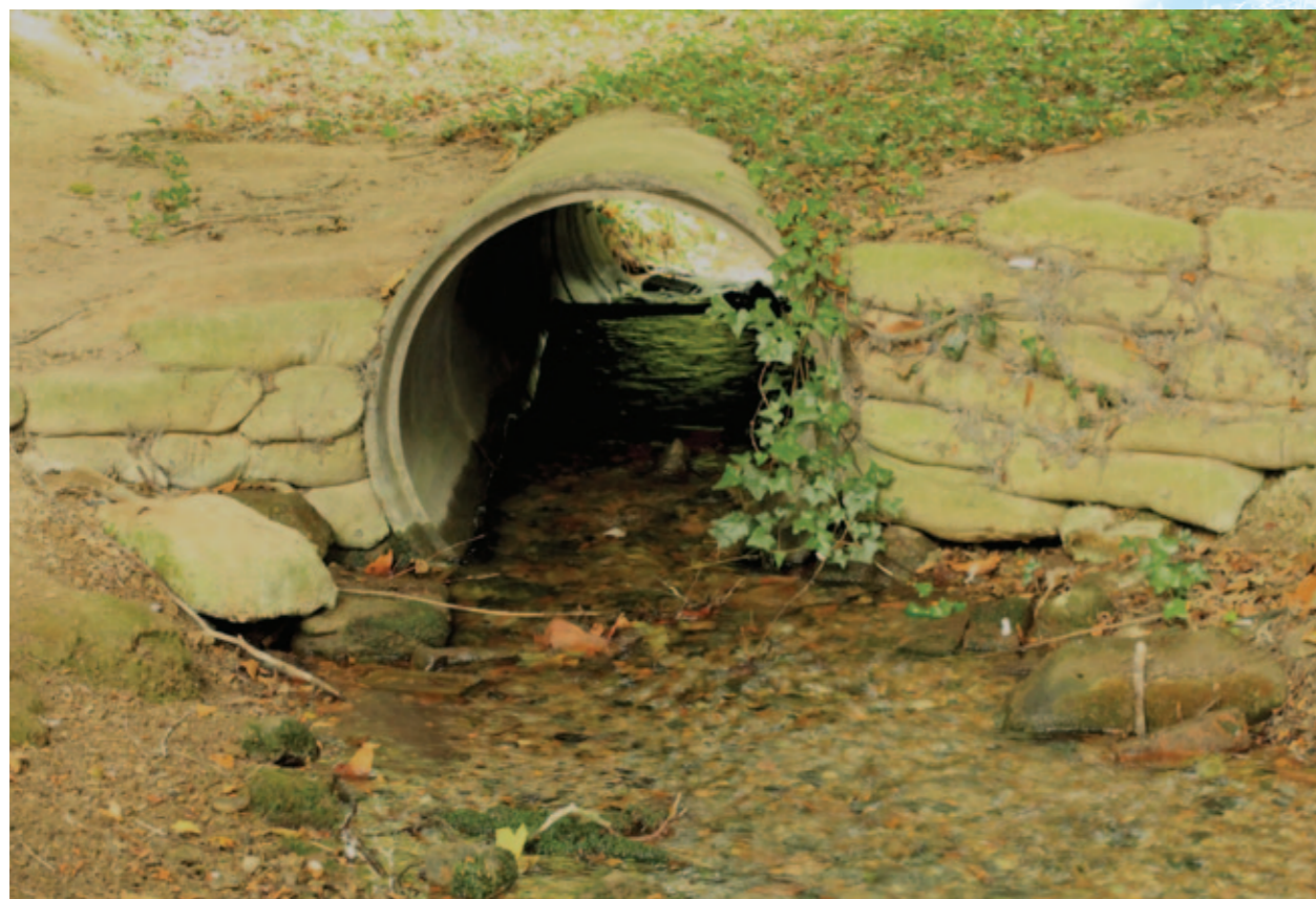
The stream flows through a culvert under the railway bridge.
